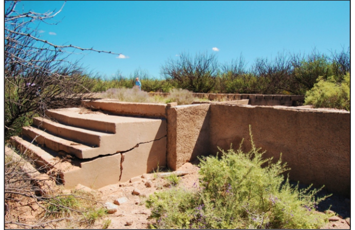
Valverde School welcomes the very infrequent visitor. The school was under construction when the flood struck in 1937. With the town abandoned after the flood, the school was never completed.
